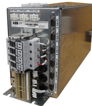
Figure 5-9: PCS100 AVC-40 Auxiliary Master Module
